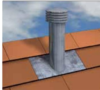
Either an older house where the existing chimney has been lined by a proprietary steel flue or a newer house with a steel flue built in. This chimney type is identifiable by a 5" (130 mm) diameter flue and a steel flue terminal.
